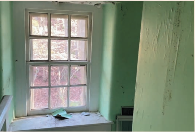
Signs of disrepair and mold in the farmhouse prior to the 2021 renovation are seen here.
